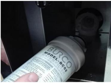
4. Twist cartridge anticlockwise to remove (some residual water may be present).
