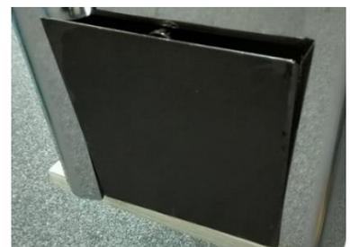
3. **Slimline Water Boiler:** Push the filter access panel, the magnetic catch releases the door, pull to open.
